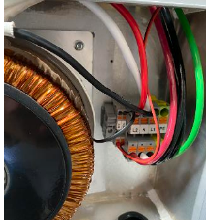
Auto-transformer connection from inverter. AC connection accepts 12 AWG min. and 6 AWG max.
